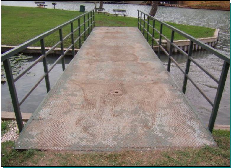
Metal foot bridge
