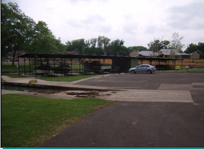
Storage facility metal awning
