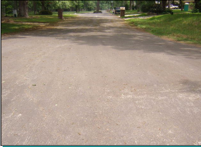
Asphalt pavement along Paseo Del Rio near Marina
