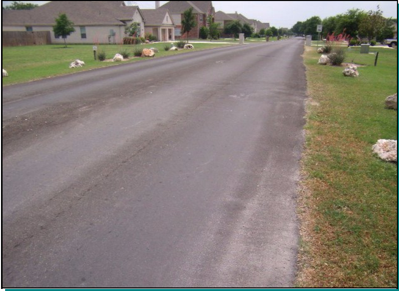
Asphalt pavement overview at entrance
