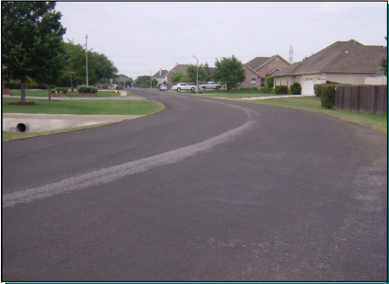
Asphalt pavement overview along Las Brisas
