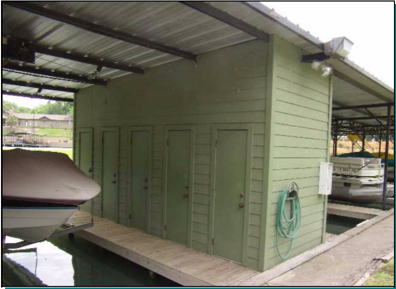
Storage facility Note: Fiber cement siding, metal doors
